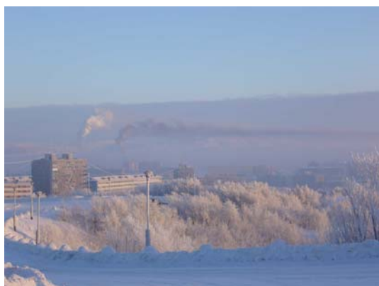
Emissions from the existing boiler house
