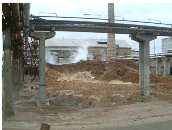
Wood waste from the production process to be used as fuel
