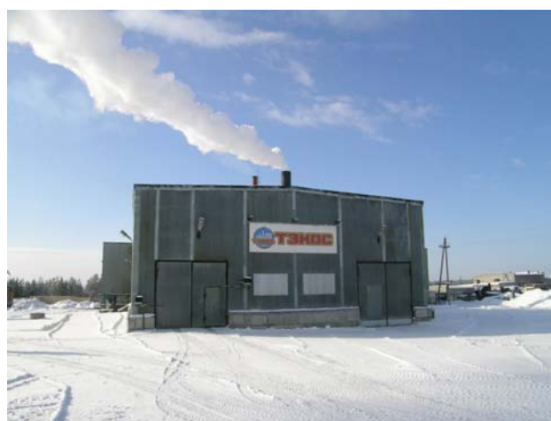
The new biofuel boiler house
