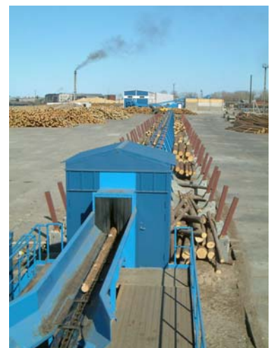
Energy intensive wet sorting line
