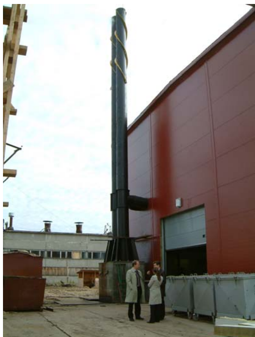
New boiler house at Tsiglomen
